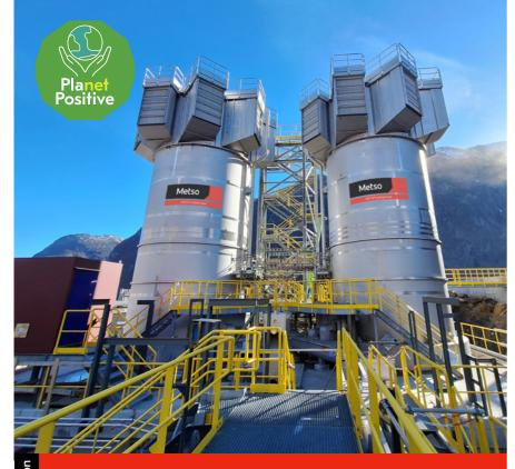
OKTOP® cooling tower provides direct-solution cooling for applications such as cooling of spent electrolyte solution and gypsum removal, in hydrometallurgical processes.
